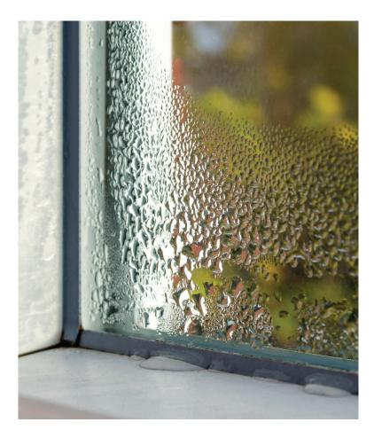
Condensation typically occurs on cooler surfaces inside the home, such as astragals, hinges, hardware and glass. These surfaces are cooler because they are closer to the outside than a wall or table, and excess moisture condensates on these surfaces. The moisture in the air is defined as humidity.
